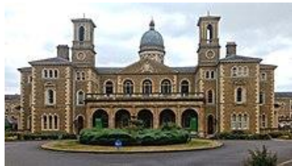
Fig.2 The main building of the former Colney Hatch asylum
